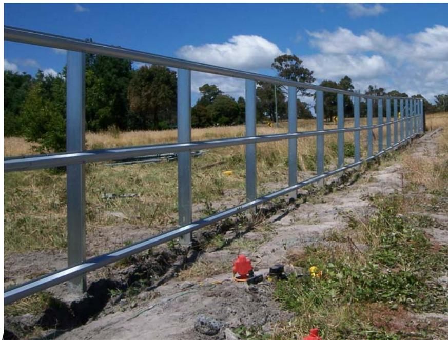
For a double sided fence a second set of rails will need to be fixed to the other side of the posts.
